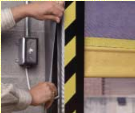
Vinyl Strip to seal the Guide Track along the edge
